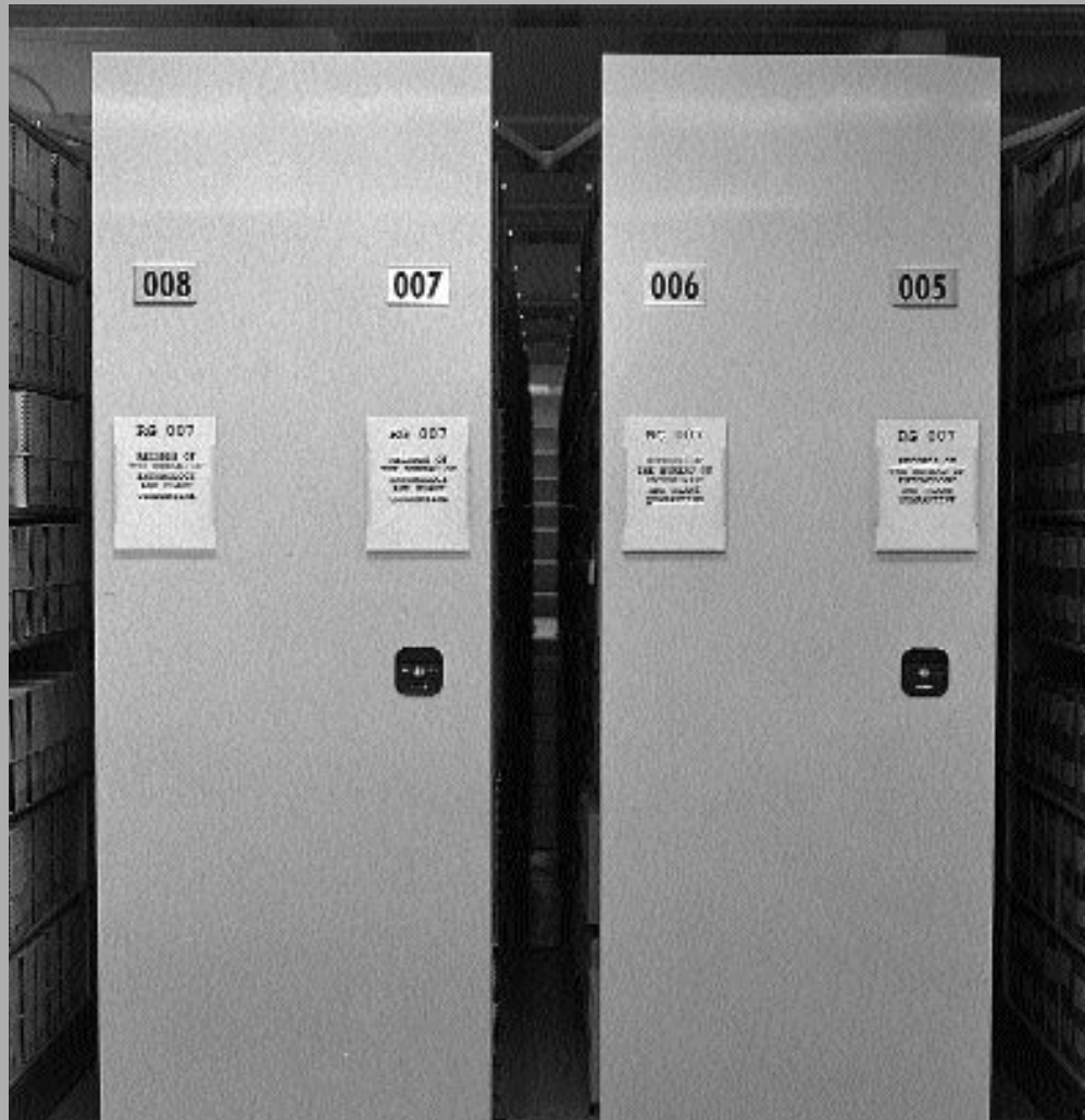
Flue spaces between the carriages reduce the time it takes to put out a fire and the amount of fire damage in a mobile shelving system.
