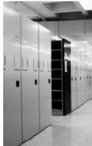
After much research and testing, NARA chose to cover the concrete floors in all stack areas with a special-formulated epoxy floor coating.
