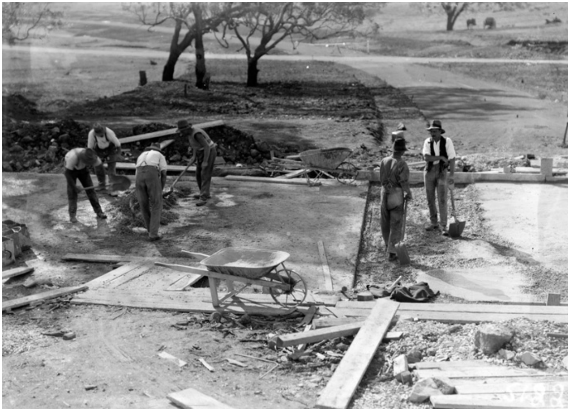
Building roads in the Federal Capital Territory, c1929. NAA: A3560, 5122
